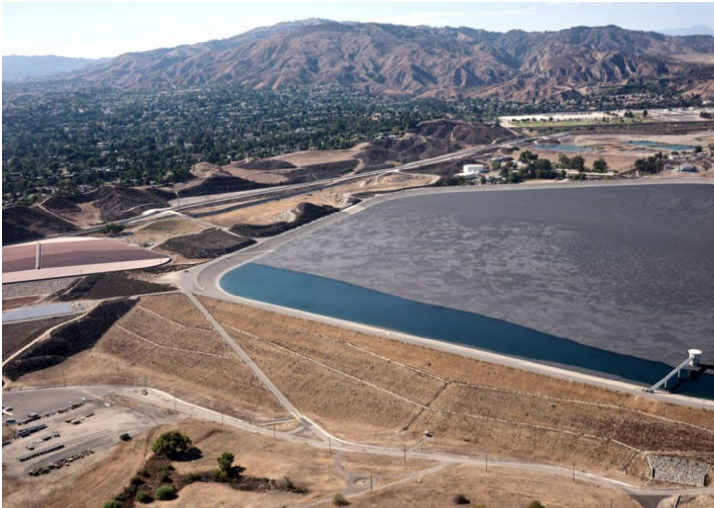
An aerial view of the Van Norman reservoir complex in Granada Hills. A project at the complex will include the construction of an ultraviolet light treatment facility on the outlet of the Los Angeles Reservoir. (Hayley Smith / Los Angeles Times)© (Hayley Smith / Los Angeles Times)
