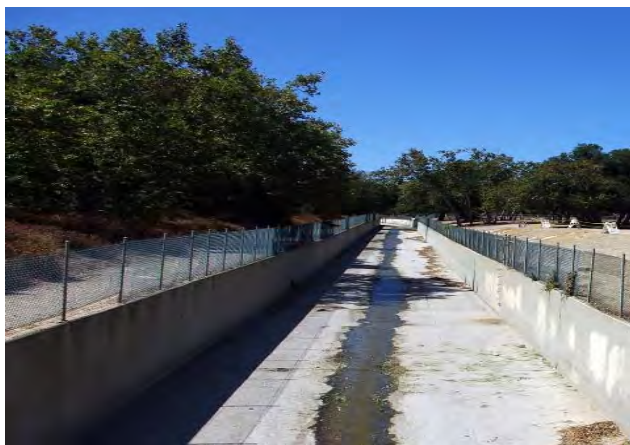
Verdugo Wash Channel
