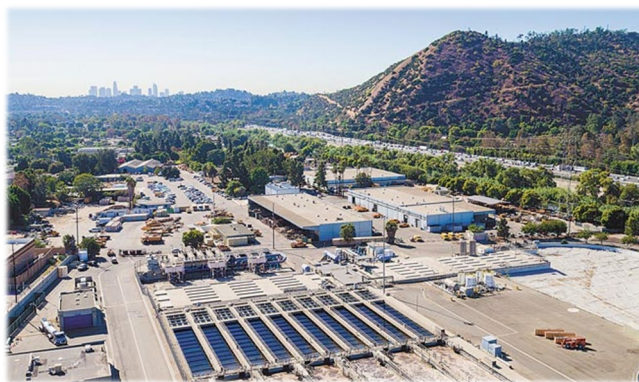
Figure 6.1: Los Angeles-Glendale Plant
