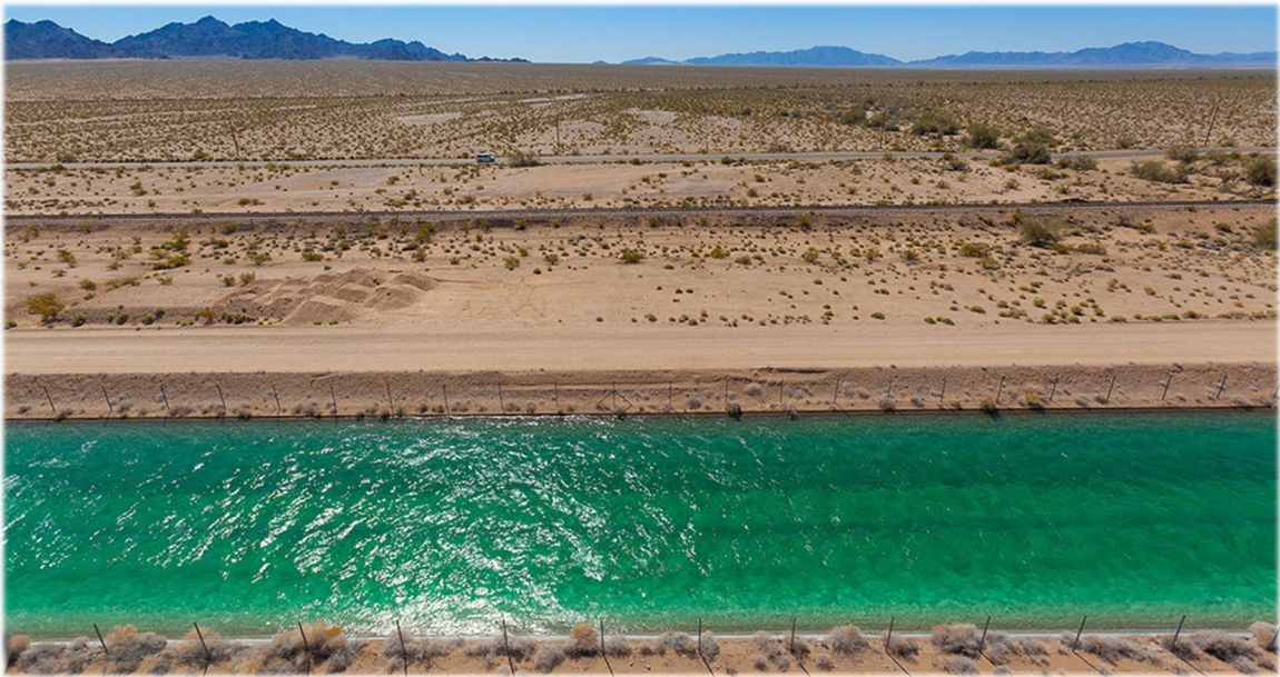
Figure 3.2: Colorado River Aqueduct
