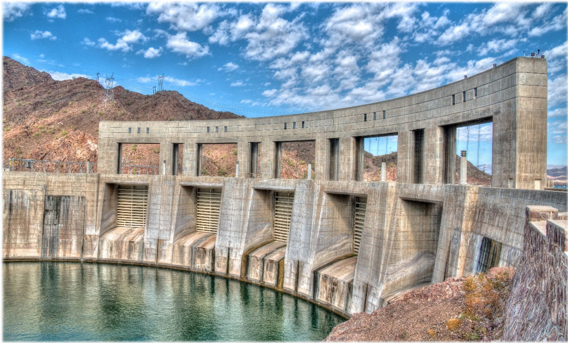
Figure 3.1: Parker Dam at Colorado River
