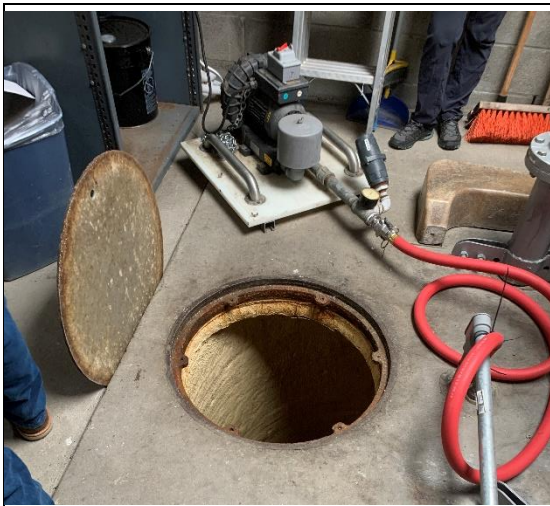
Figure 1: Manhole opening inside of pump station building
