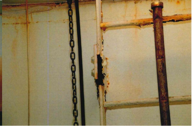
Edmund No. 2 – 2020 Spliced Connection at Ladder
