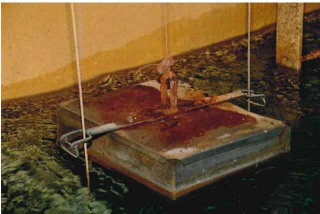
Edmund No. 2 - 2020 Liquid Level Indicator
