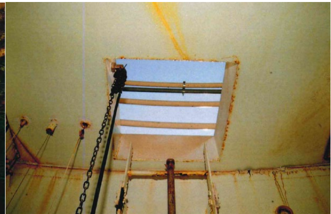
Edmund No. 2 - 2020 Roof Hatch
