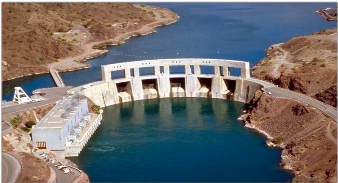
Figure 3-1: Parker Dam at Colorado River
