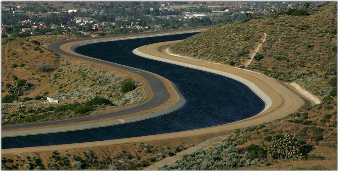
Figure 3-4: California Aqueduct or "SWP"
