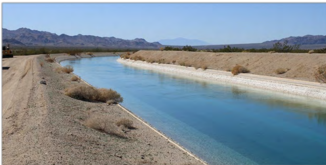
Figure 3-3: Colorado River Aqueduct
