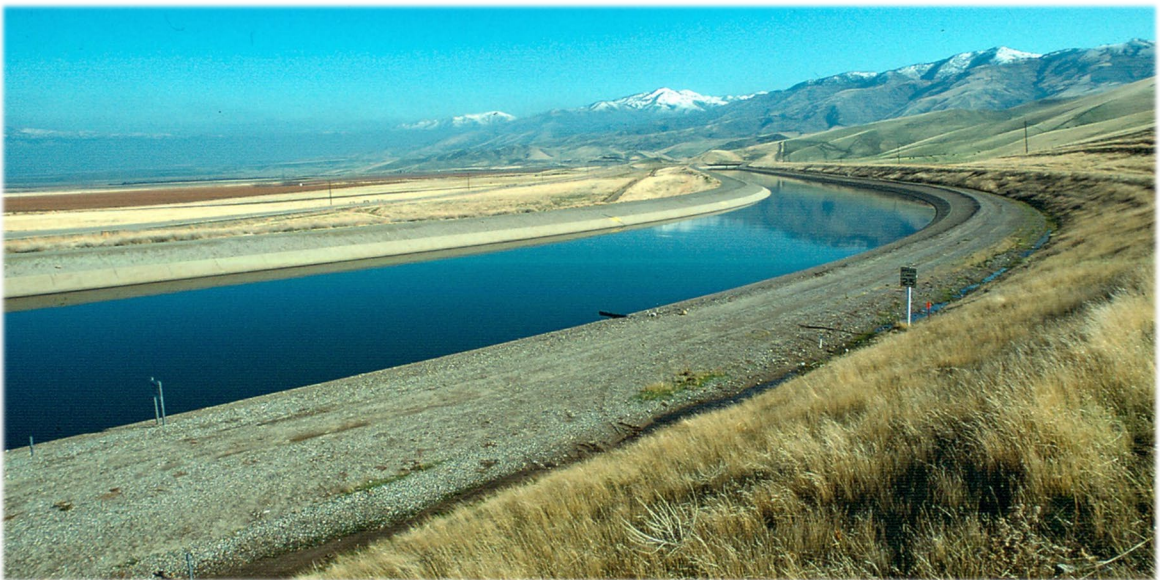
Figure 3.3: California Aqueduct or “SWP”
