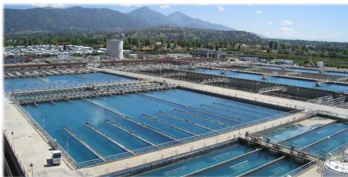
Figure 3.9: MWD's Weymouth Treatment Plant Provides a Safe Supply of Water
