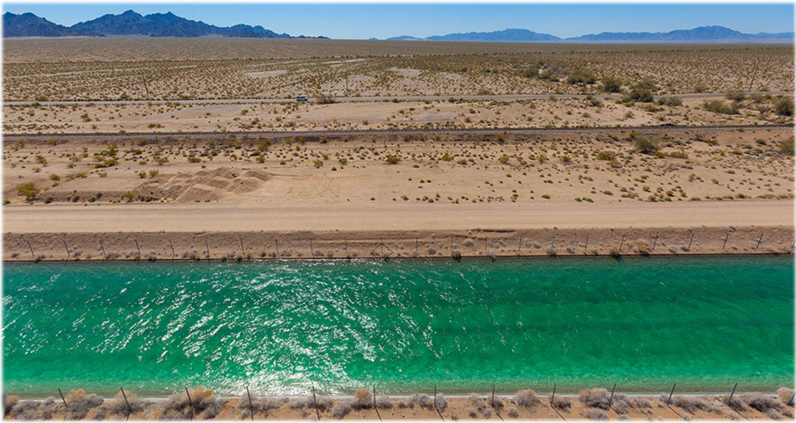
Figure 3.2: Colorado River Aqueduct
