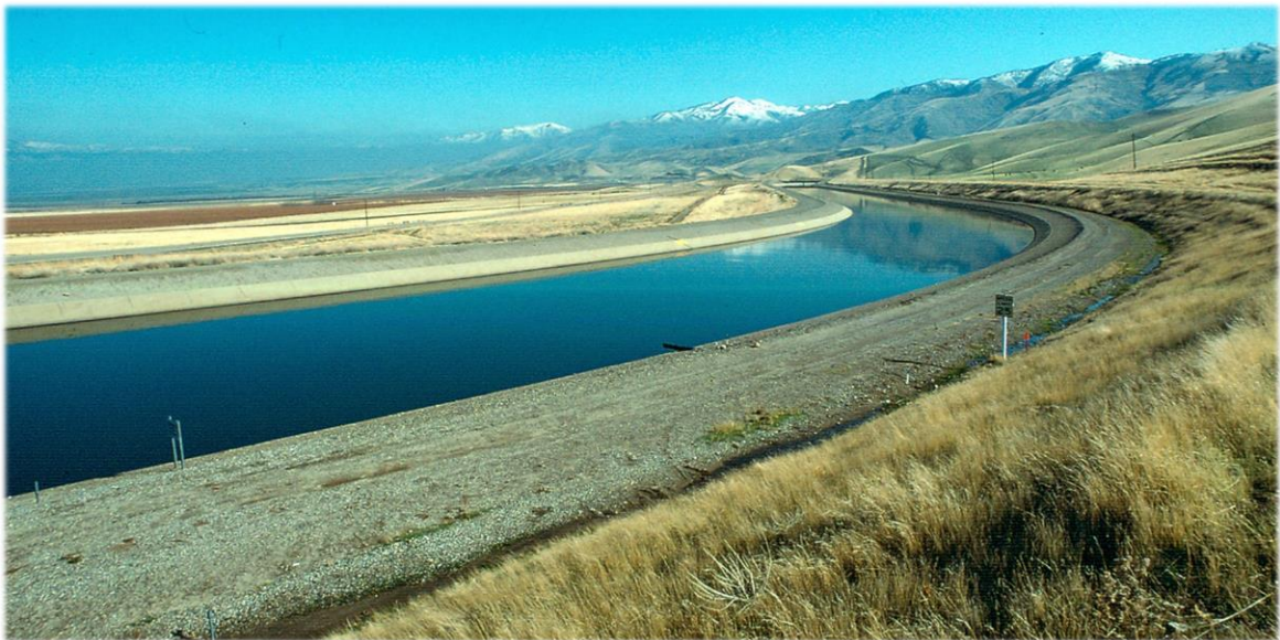
Figure 3.3: California Aqueduct or “SWP”
