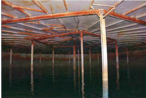
Oak Creek #1 - 2011 Above the water line
