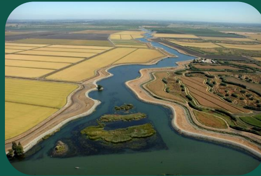
State Water Project
