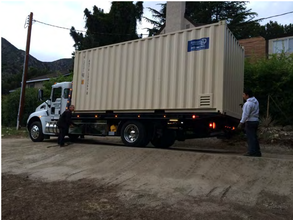
Edmund #1 Site – Delivery of Storage Bin
