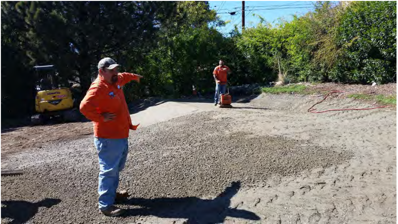
Edmund #1 Site – Compacting Base Material for Level Pad
