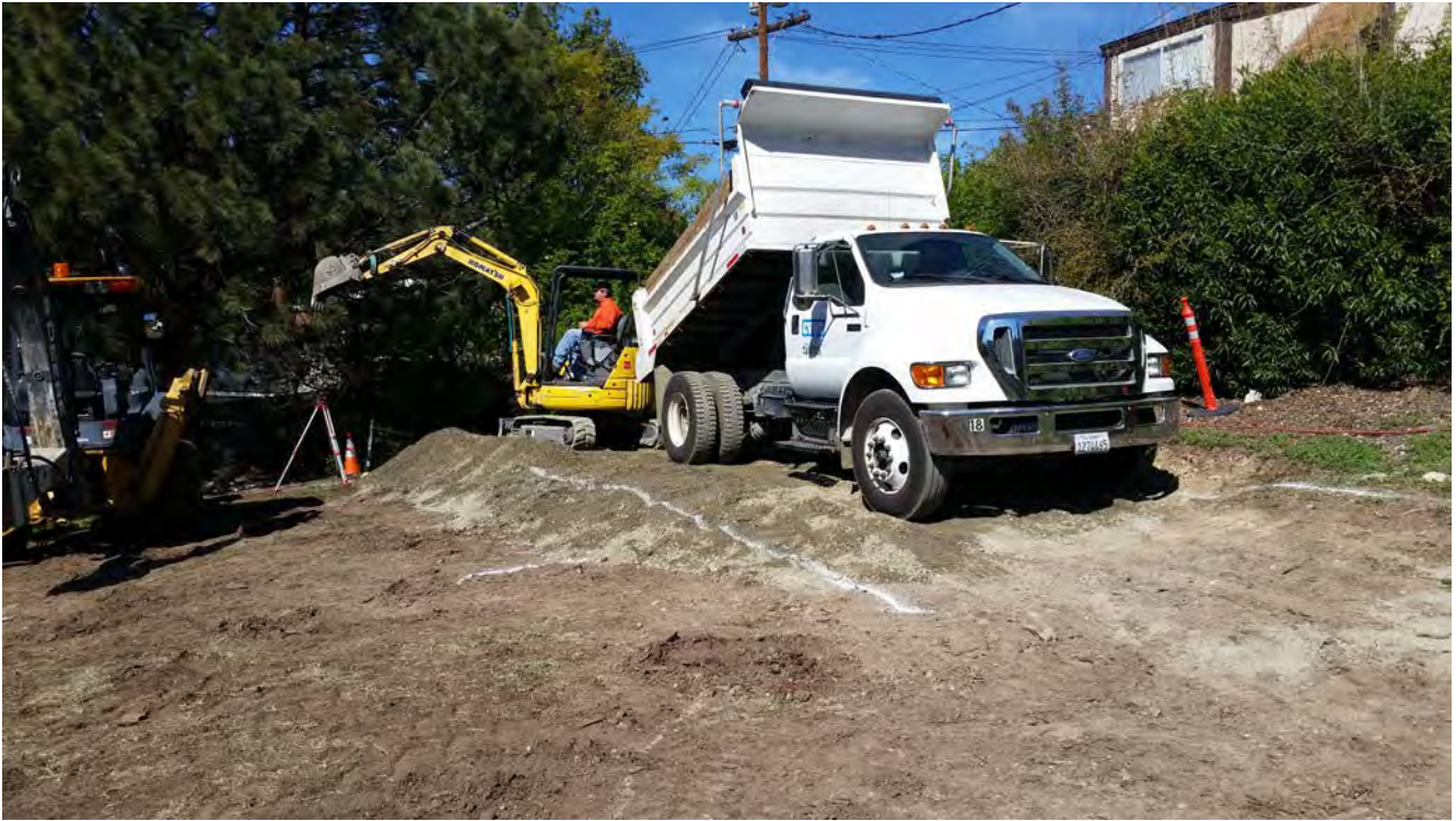
Edmund #1 Site – Unloading Base Material
