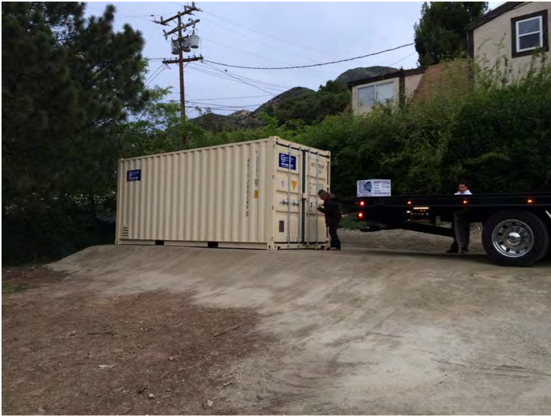
Edmund #1 Site – Storage Bin in Place
