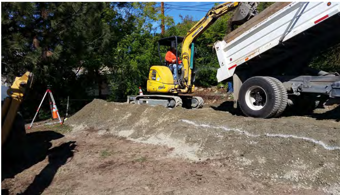
Edmund #1 Site – Grading & Filling with Base Material
