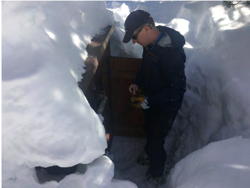
Photo: Snow is so deep at the equipment shed at the Slide Mountain SNOTEL site that hydrologist Jeff Anderson had to dig a pit just to get to the door.
