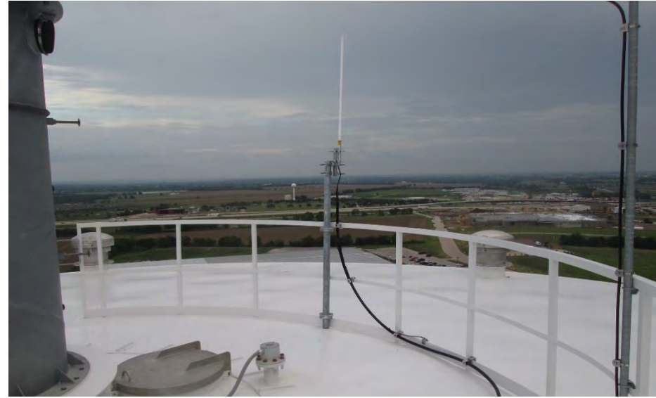
Tank Rail-Mounted Collector with Short Mast
