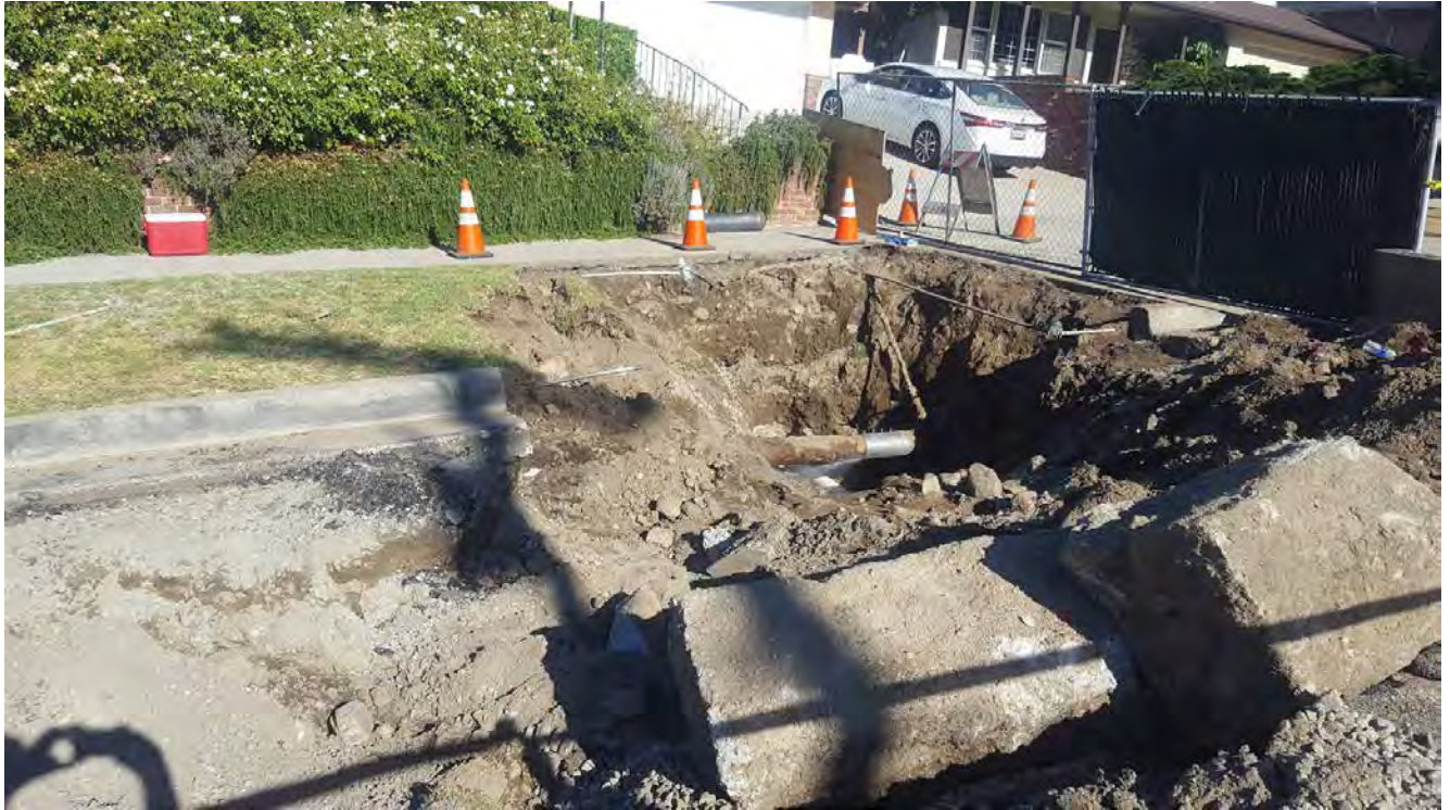
Temporary Pipe Repair
