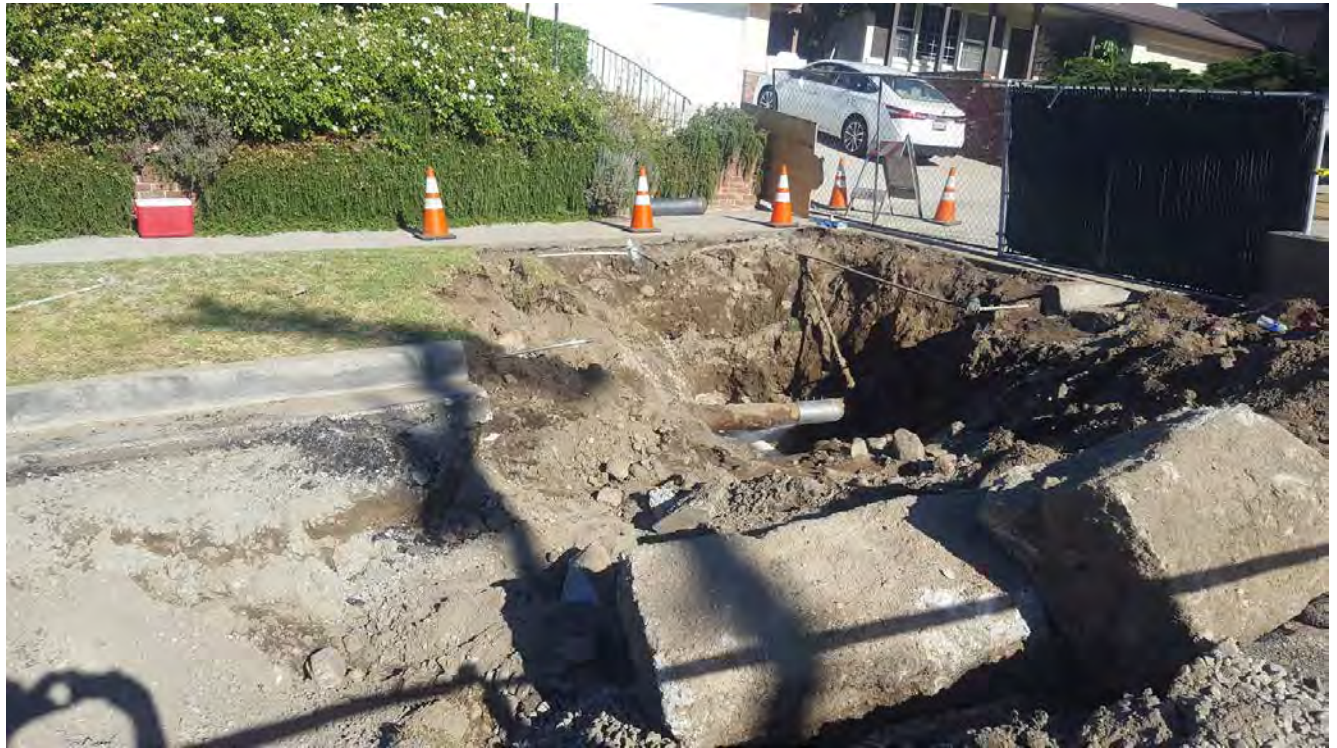
Temporary Pipe Repair
