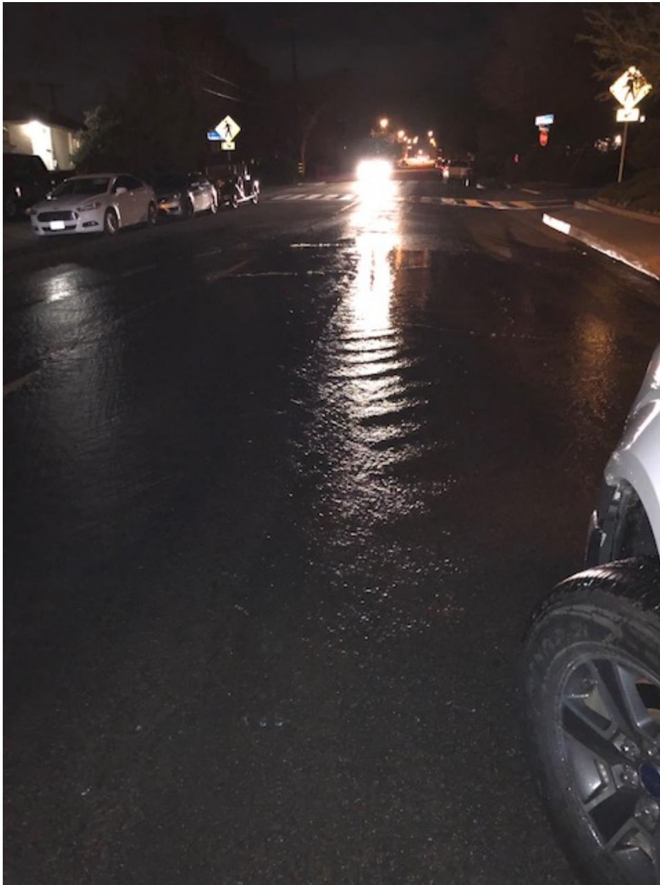
Water Main Break – Rosemont & Prospect
