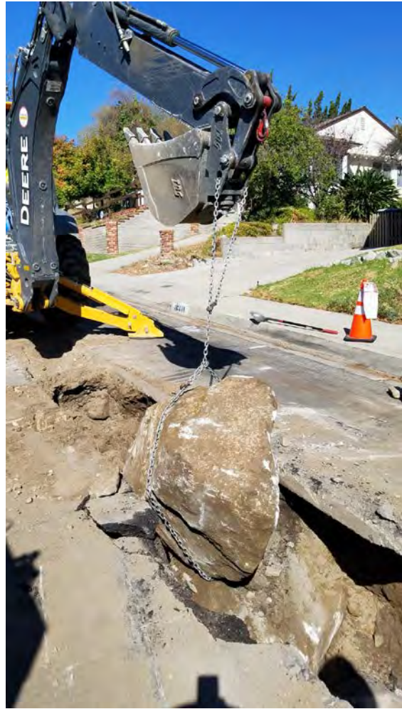
E-1002 – Boulders Discovered While Excavating on the 3300 Block of Brookhill
