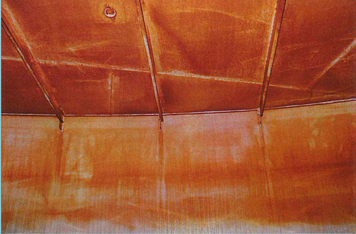
Oak Creek No. 1 – Interior Roof
