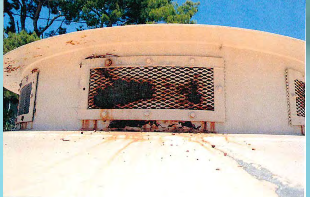
Oak Creek No. 2 – Vent
