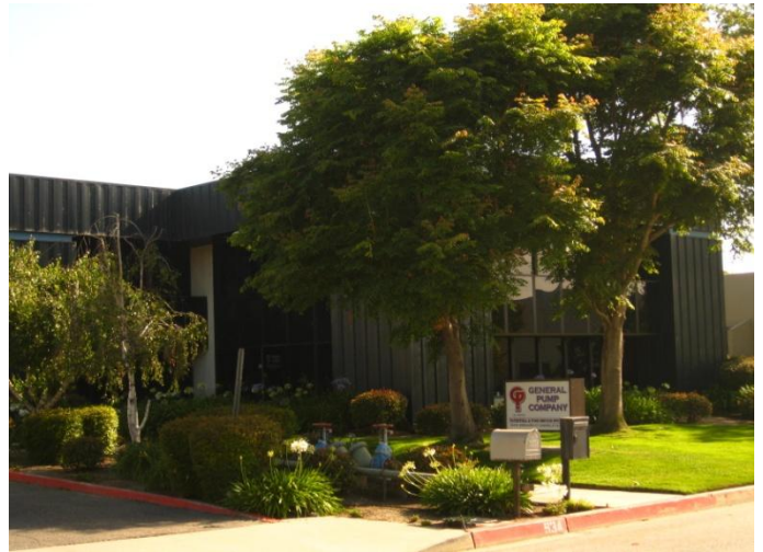
Camarillo Pump Engineering Center
