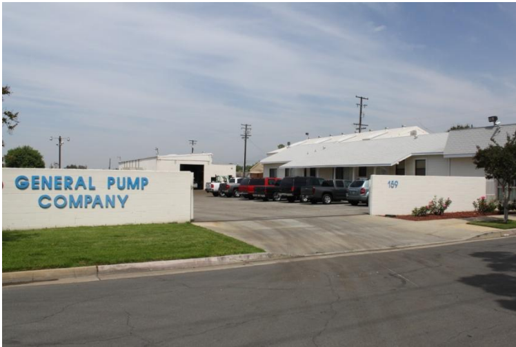
San Dimas Pump Engineering Center
