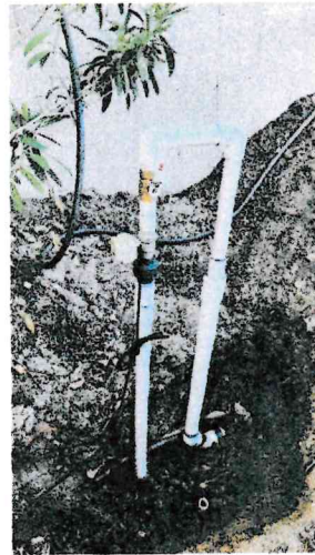
PIC 6. Motorized Valve Install
