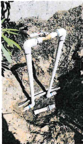
PIC 5. Ball Valve Install
