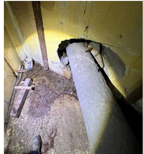
Figure 1: Interior of the Rosemont Overcrossing
