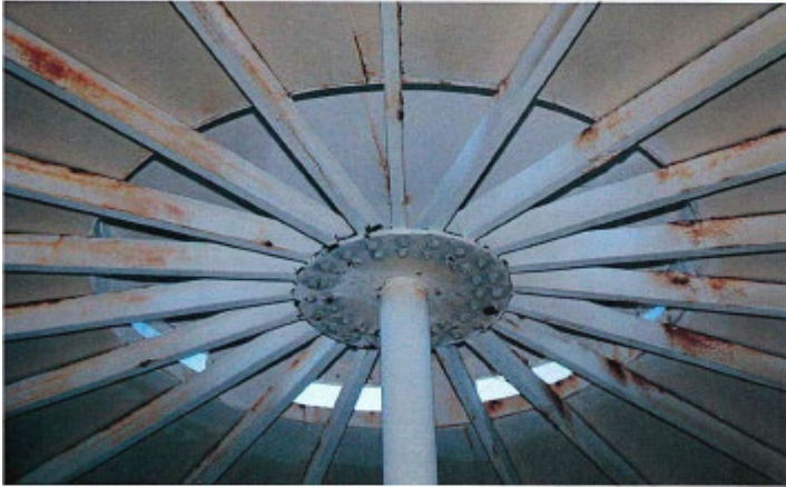
View of underside center vent cover
